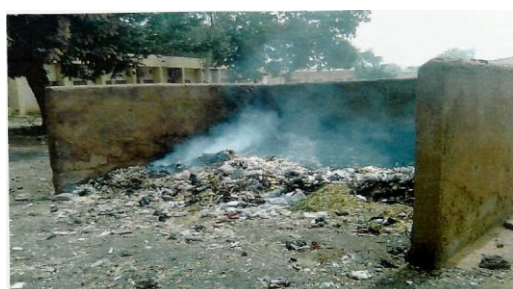
Plate ii: Walled incinerator for burning medical waste
