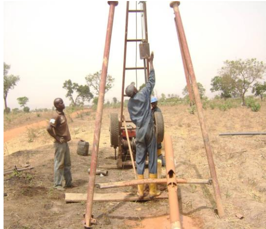
Plate 1 A trip hammer attached to a winch cable of the rig
