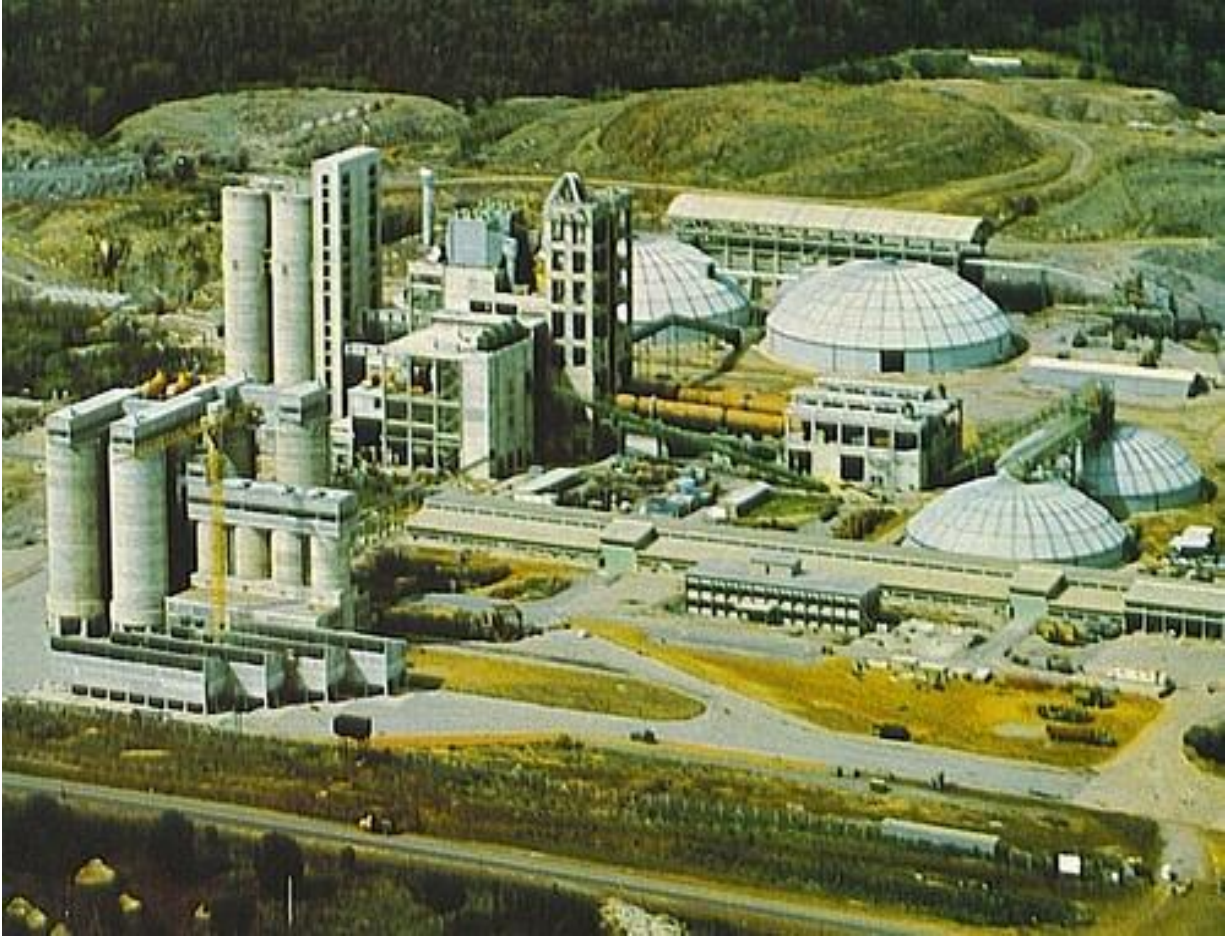
Plate V. Pollution from Benue Cement Company at Yandev near Gboko
