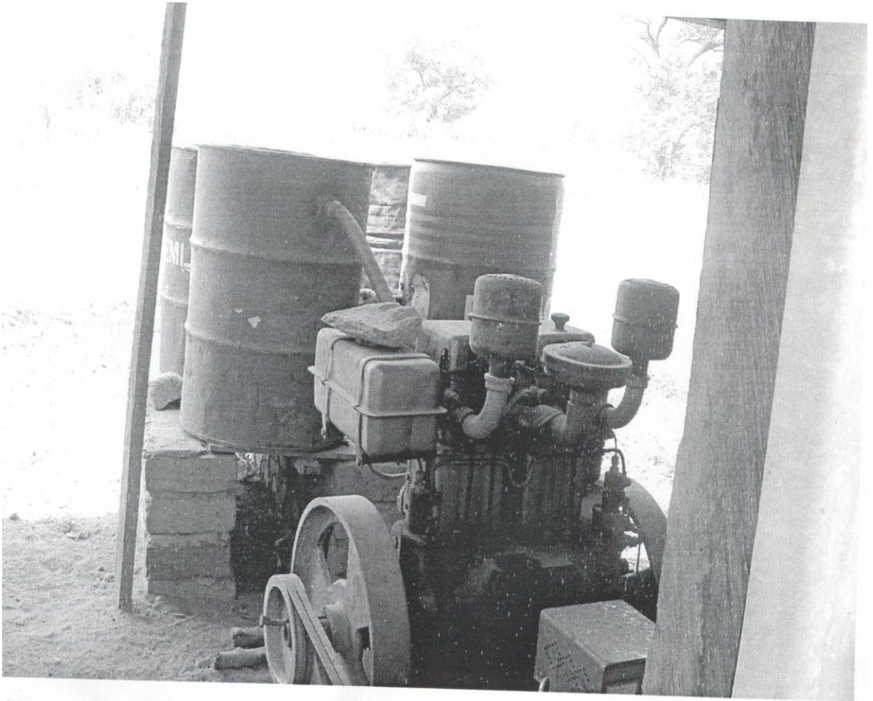
Plate XV: A Power Generator Set Bought for General Hospital Oju.
