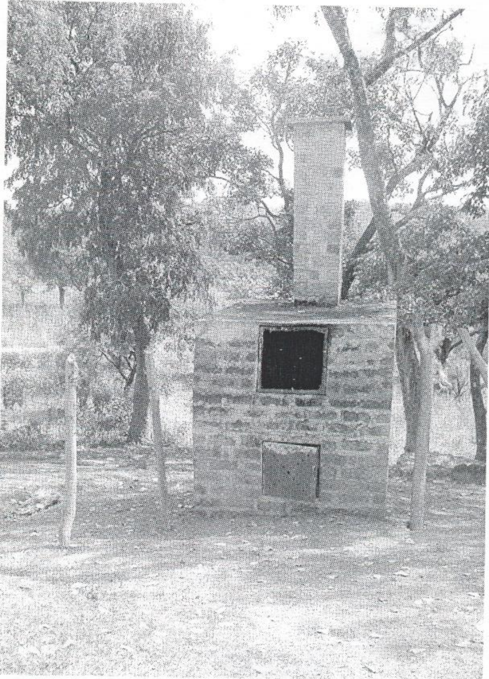
Plate XI: An Incinerator Constructed at General Hospital Gboko.
