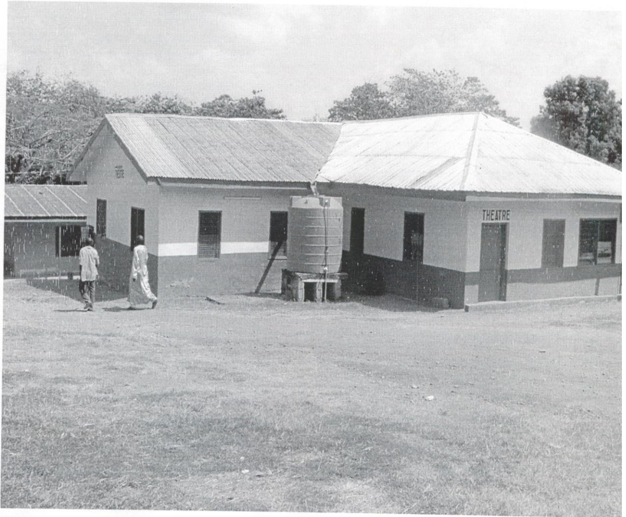
Plate IX: A Renovated Theatre Block at NKST Hospital Mbaakon, Vandeikya LGA.
