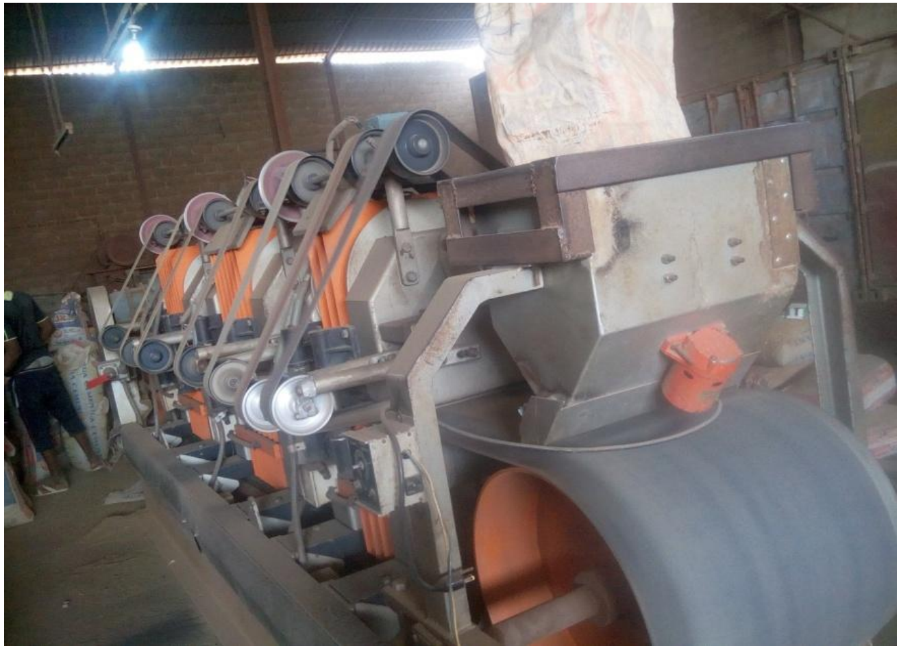
Plate 1: The Conveyor Belt under consideration
